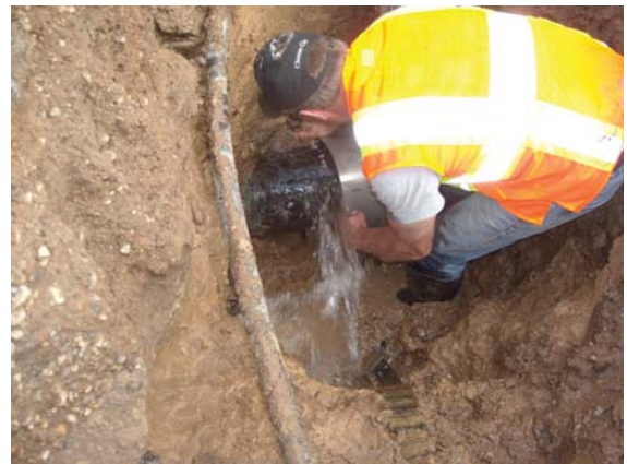
(Failure of a 35-year-old ductile iron pipe)
